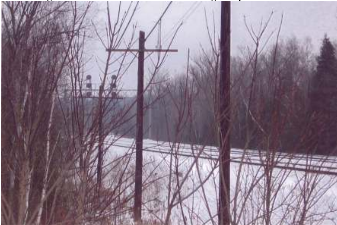
Figure 4. Railroad and Phone Lines Along Campbellville Road
